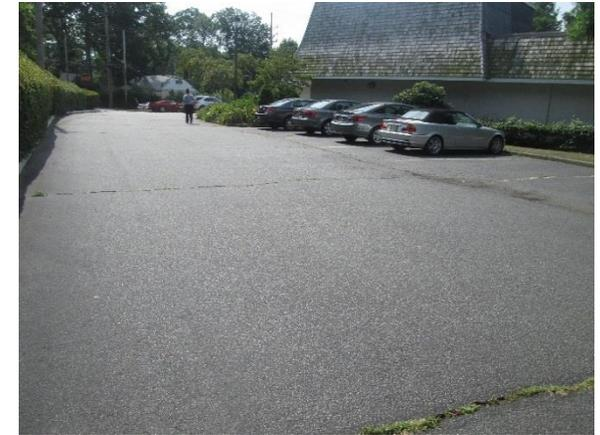
Runoff from the parking lot is directed to the stream behind the building. Parking spots can be replaced with porous asphalt to capture and infiltrate stormwater. The installation of a rain garden adjacent to the building can capture, treat, and infiltrate roof runoff. A preliminary soil assessment suggests that the soils have suitable drainage characteristics for green infrastructure.
