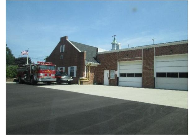
Runoff drains from the fire company to the highway. A rain garden can be installed adjacent to the building to capture, treat, and infiltrate roof runoff. Cisterns can be installed behind the building to harvest rainwater. The water can be used to wash the emergency vehicles on site. A preliminary soil assessment suggests that the soils have suitable drainage characteristics for green infrastructure.
